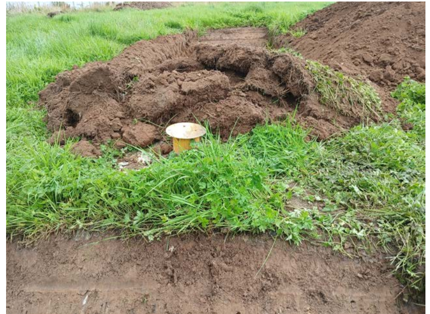
Plate 4: Area skipped over in Trench 1, due to water services, looking east.
